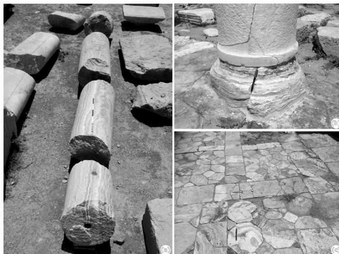
Fig. 3 Banded travertine blocks used for different purposes a) columns, b) column basement and c) paving.
