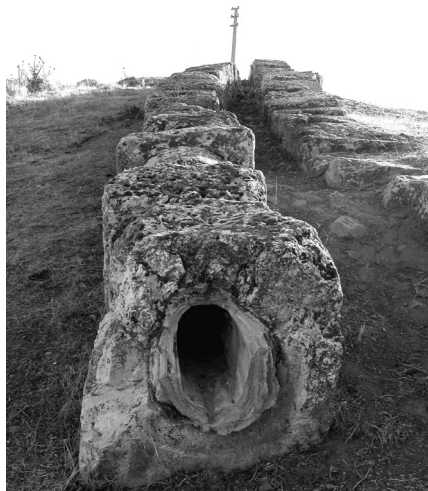
Fig. 19 Twin travertine pipes near Eskihisar
